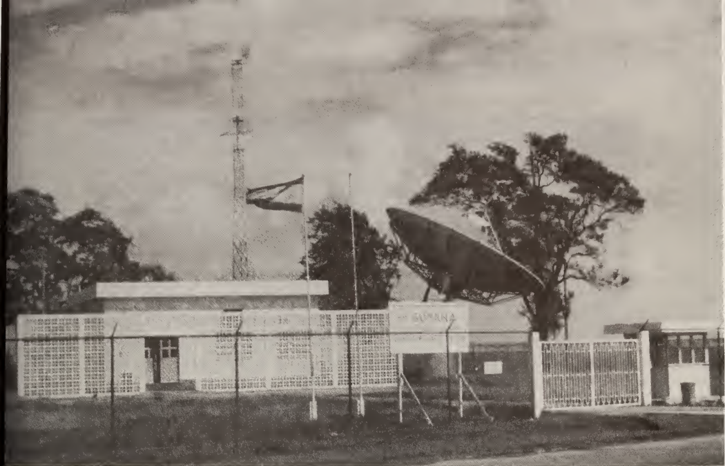
Ground satellite station at Georgetown Courtesy Embassy of Guyana, Washington
