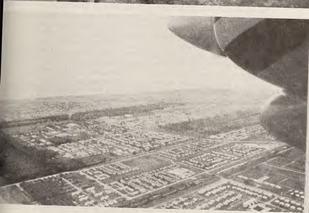
Aerial view of the low-lying coast with its Dutch-built seawalls Aerial view of Georgetown showing the layout designed by the Dutch, mostly on a grid pattern Courtesy Embassy of Guyana, Washington
