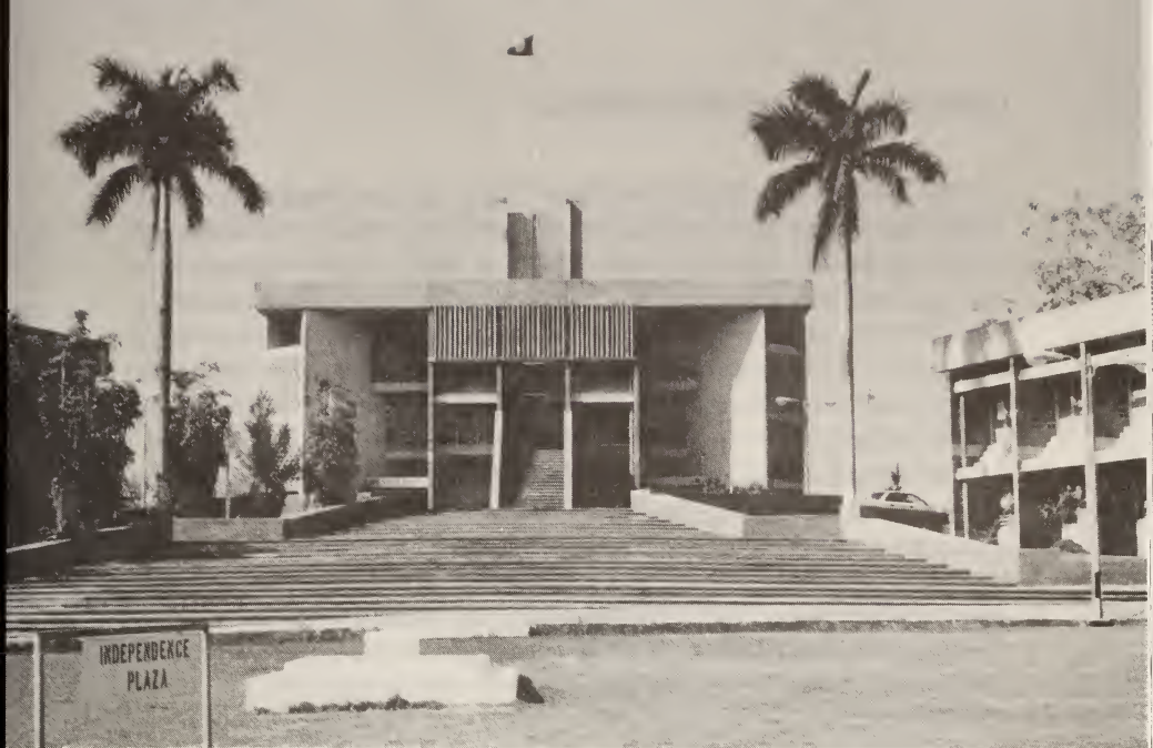
National Assembly building, Belmopan Courtesy Steven R. Harper
