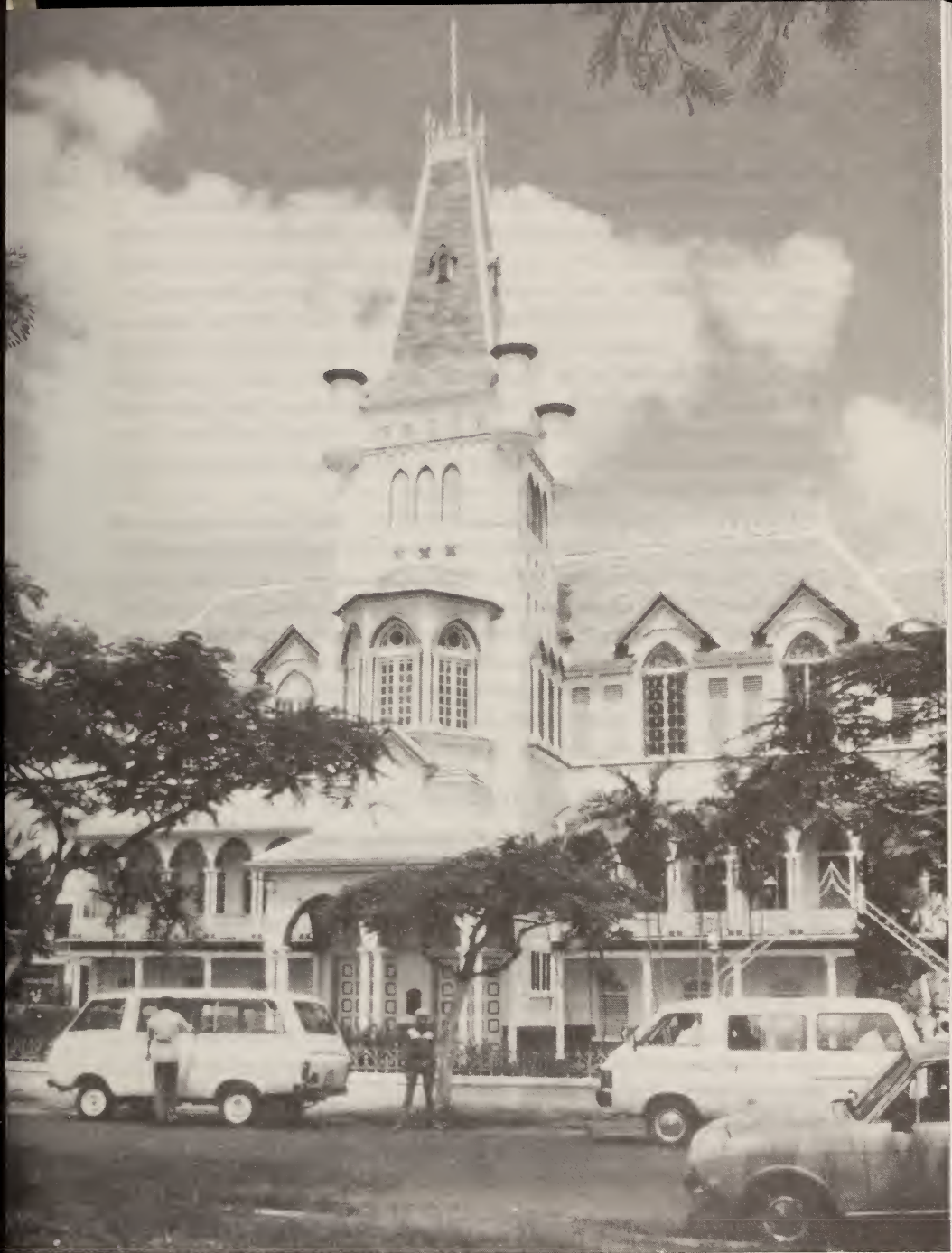
City Hall, Georgetown. Completed in 1889, it is one of the finest examples of Gothic architecture in South America. Courtesy Embassy of Guyana, Washington
